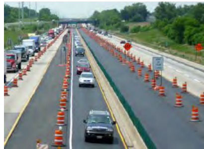
Delineate traffic lanes during resurfacing work
